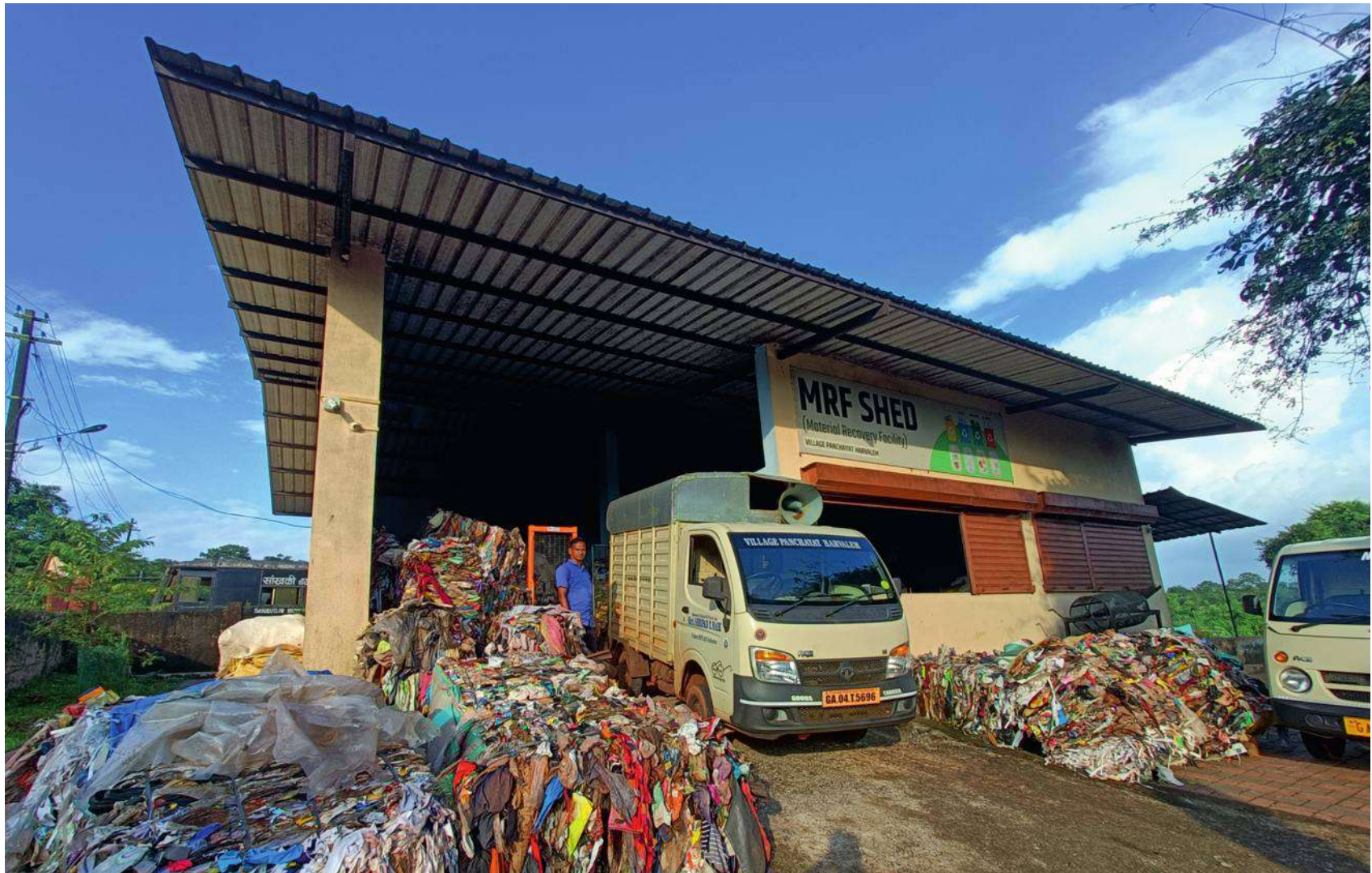
Material Recovery Facility(MRF)
